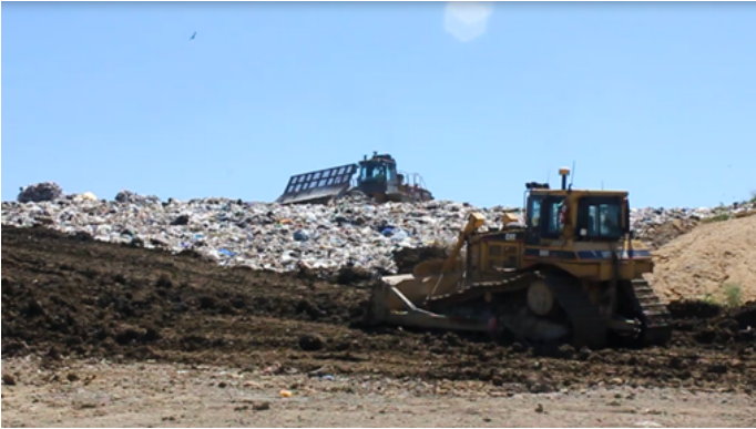
This photo shows daily cover of soil being applied.
