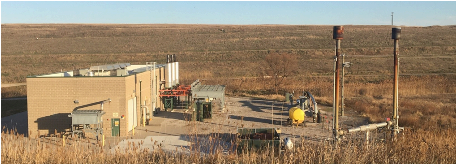
This photo shows one of two Methane Recovery Facilities at Metro Park East landfill.
